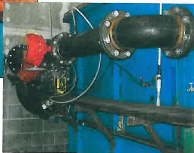
Figure 9: Floc Basin Inlet Pipe (after replacement)
