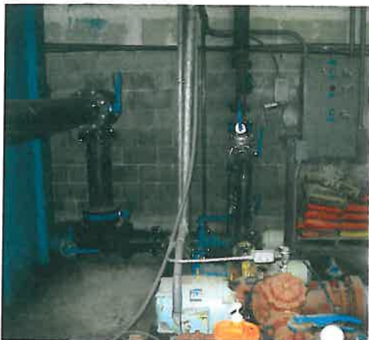
Figure 6: NEW Piping out of the Floc Basin
