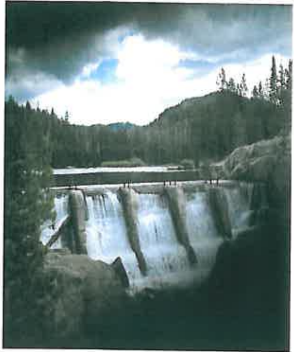
Figure 10: Herring Creek Reservoir Dam
