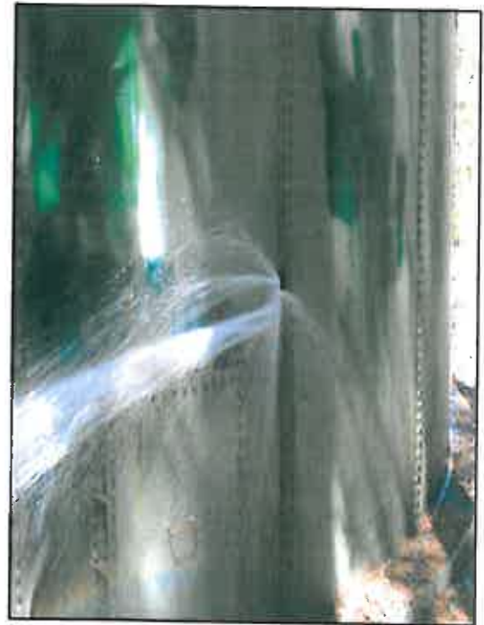
Figure 2: Lower Dymond storage tank
