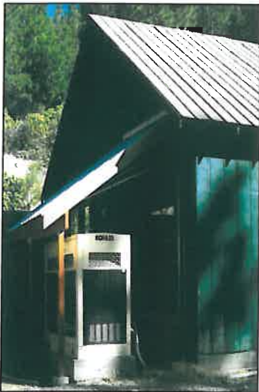
Figure 5: Standby generator at the treatment plant
