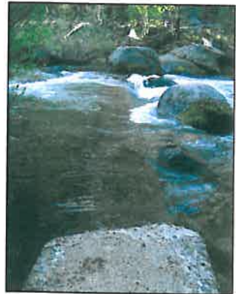
Figure 1: Herring Creek Intake
